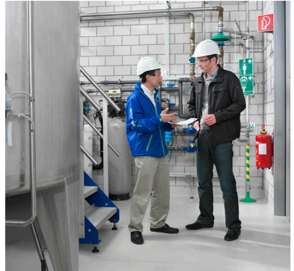
Expert, manufacturer's assessment of equipment our technicians are factory-trained to inspect and document the condition of your METTLER TOLEDO intrinsically safe weighing equipment. We use procedures and documentation consistent with the IEC standard Explosive atmospheres – Part 17: Electrical installations inspection and maintenance.
